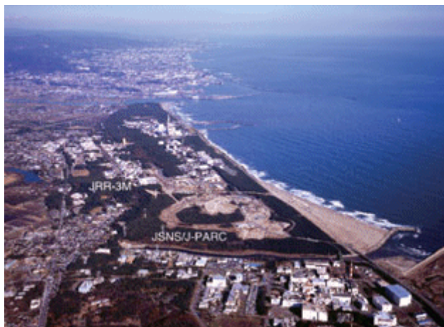
Fig. 3-3-2 An aerial photograph of the construction site of J-PARC in Tokai Research Establishment of JAERI directly facing the Pacific Ocean. JRR-3M reactor currently operational and JSNS under construction are located within 1km. Photo taken from the right hand side (south) of Fig. 3-3-1.
