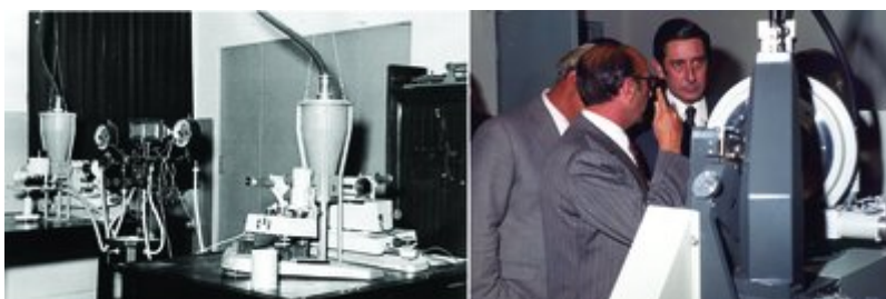
Left: Weissenberg cameras and X-ray tubes used in Madrid during the 60s. Right: The first automated 4-circle diffractometer (PW1100) installed in Spain, Madrid, in 1973.
